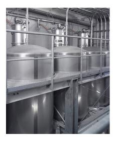
Dilute phase conveying is also the most economical mode in many cases because the equipment used in these systems are typically easier to clean and maintain. Dense phase systems typically require higher pressures, and vessels built to withstand these pressures must meet codes set by the American Society of Mechanical Engineers (ASME). These heavy vessels are more difficult to take apart and inspect (and therefore clean) due to the amount of extra flanges, bolts and fasteners required.
