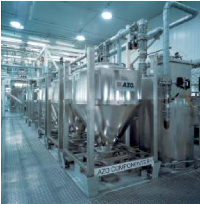
The DOSITAINER®: transportation, storage and metering plus product changeover without residue.
